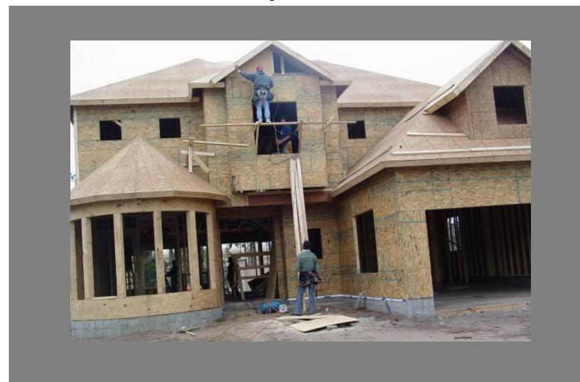
A worker is working from a carpenters' scaffold that has no guardrail, extends too far beyond either end, and is not wide enough.
