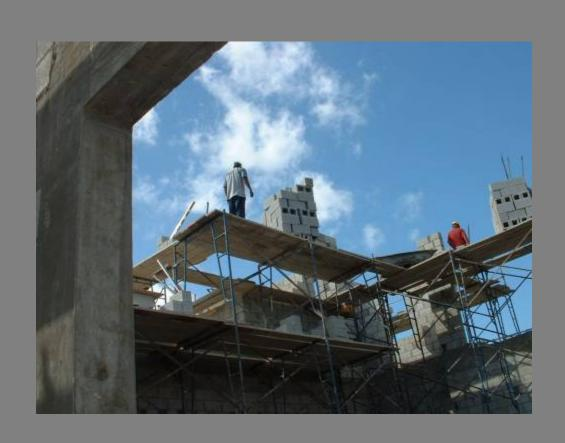
Lack of fall protection for workers on fabricated frame scaffolds.
